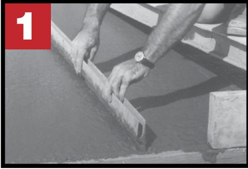
**STEP ONE:** A straight edge or other type of thin bladed material can be used to separate the aggregate in freshly poured on-grade slabs. The aggregate can be separated by using a back and forth motion approximately 2" deep.
